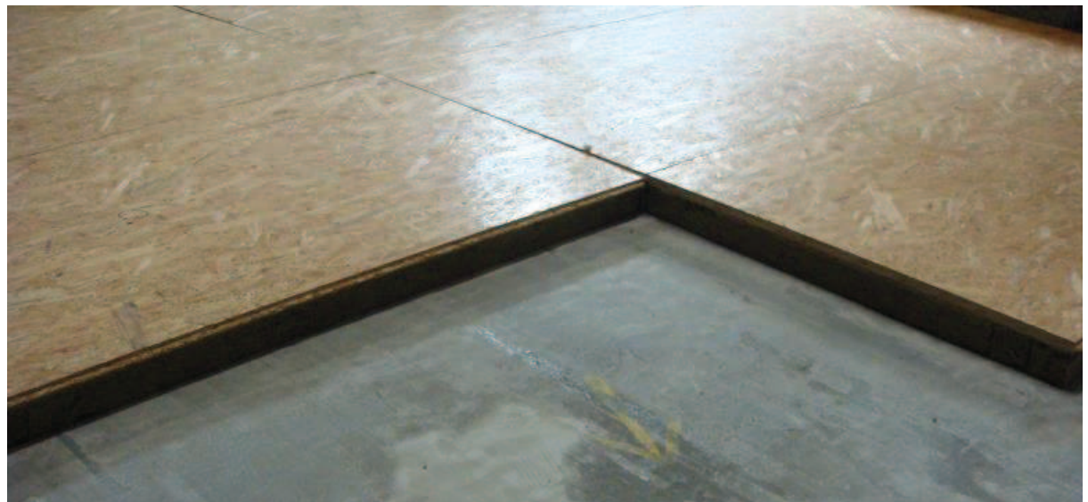
product during mounting in floor test opening
